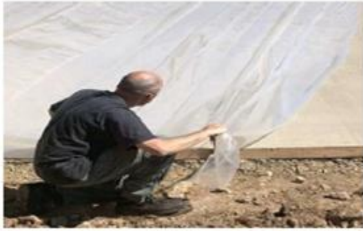
Fig. 14 Concrete curing
