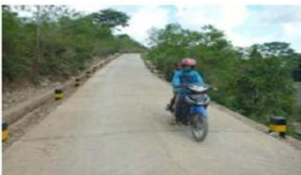
Fig. 7 Plum Concrete Pavement
