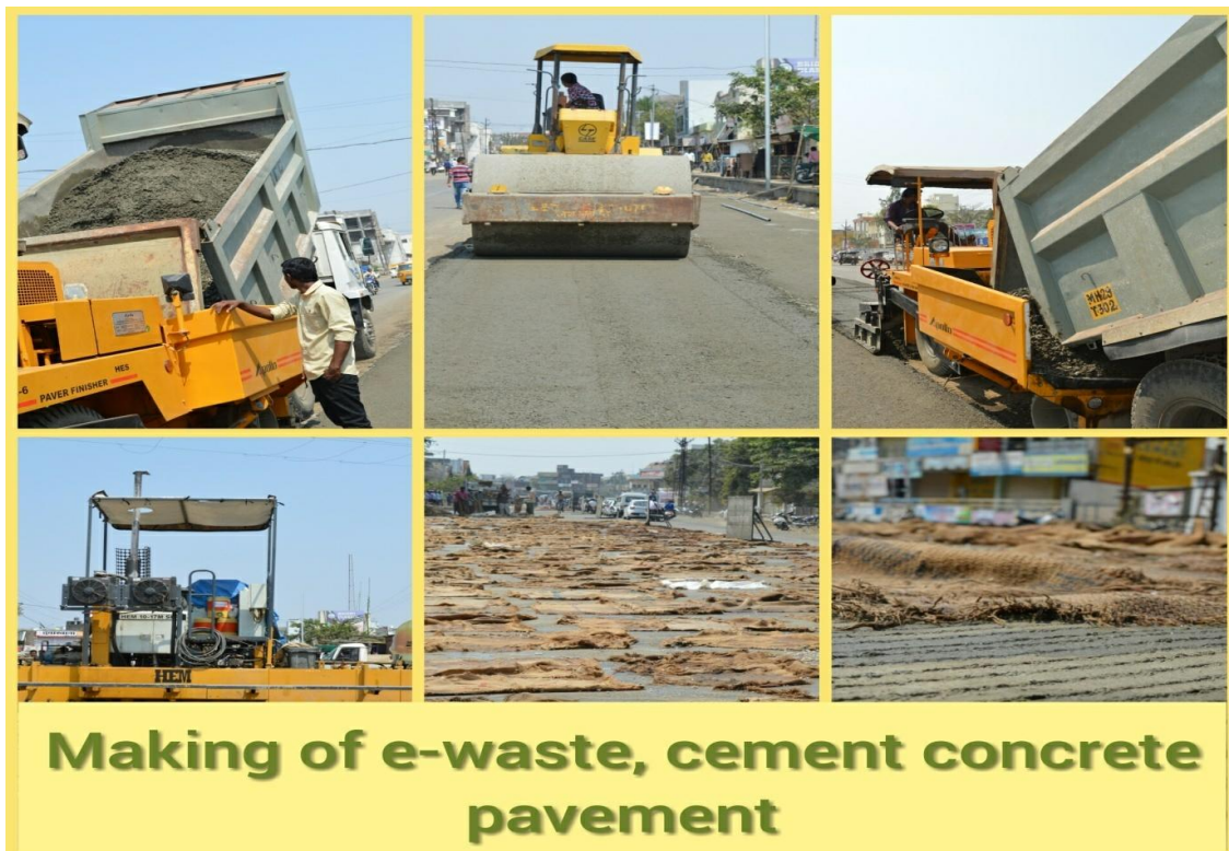
Fig 6: Processes involved in making e-waste and cement concrete pavement
