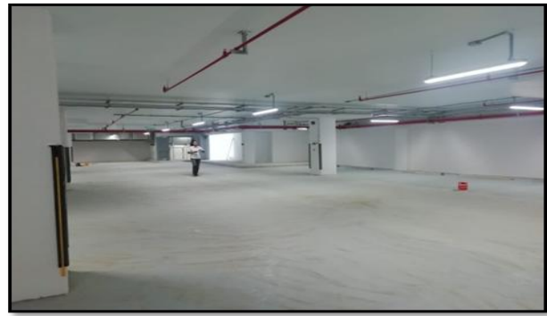
Fig. 4: PDR testing environment in an underground garage
