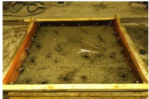
Figure 8: Partial Casting of Concrete into Flat Plat of the Wood Forms
