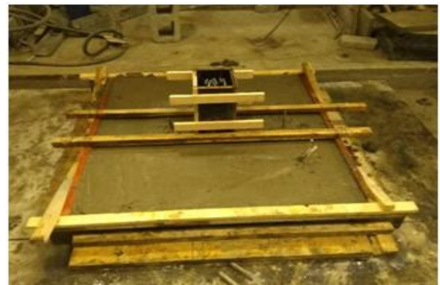
Figure 9: Fully Casting of Concrete into Flat Plat of the Wood Forms
