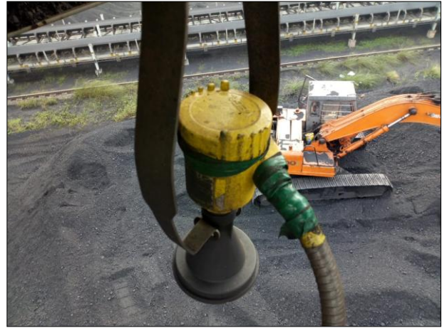
Fig. 4: stock pile sensor in GPL
