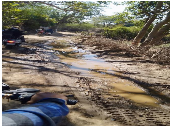
Fig. 4: Improper Drainage Condition
