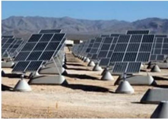
Figure 2: solar power plant
