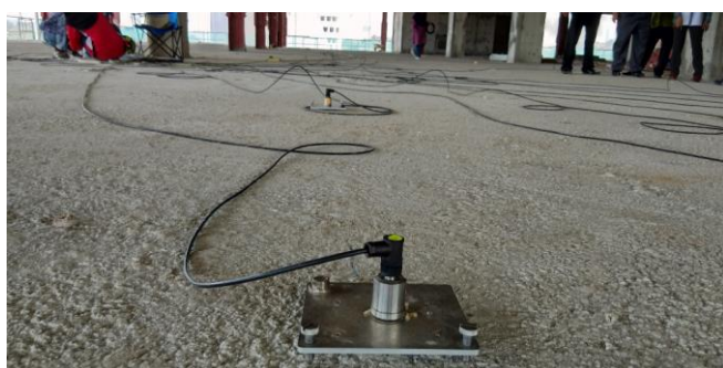
Fig. 5 Accelerometer setups at floor area A.
