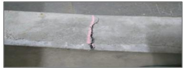
Fig. 2. Specimen after the failure in flexure test
