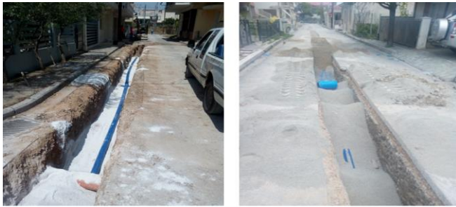
Fig. 3. Installation of new polyethylene water pipe, PE-16atm.
