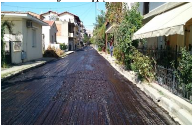
Fig. 5. Pavement adhesive application, district of Agios Georgios, Larissa, Greece.
