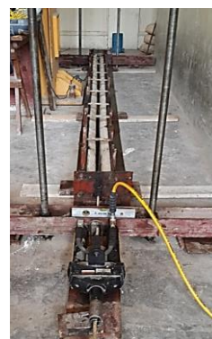
Fig. 8. Casting and Prestressing Setup
