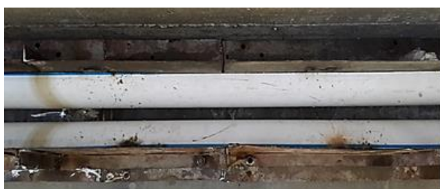
Fig. 5. Formwork of Slab Mold
