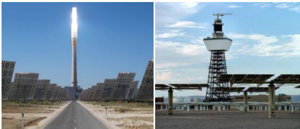
Fig. 1 A) GEMASOLAR Thermosolar Plant [29]. (B) Solar-Two plant, Source KJKolb/CC-BY-SA-2.0
