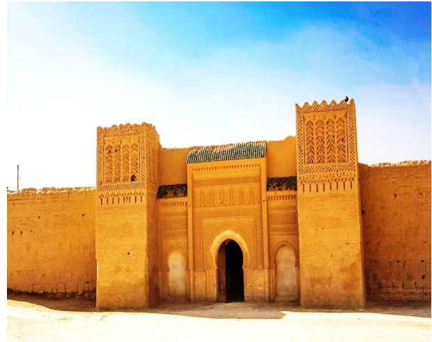
Fig.1. Overview of the Studied Building
