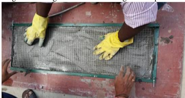
Fig.4 placing of wire mesh during casting
