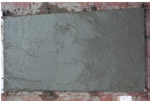
Fig.5 Ferrocement panel after finishing
