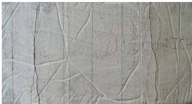
Fig. 30 Crack pattern of 2% inhibited single layer crimped panel
