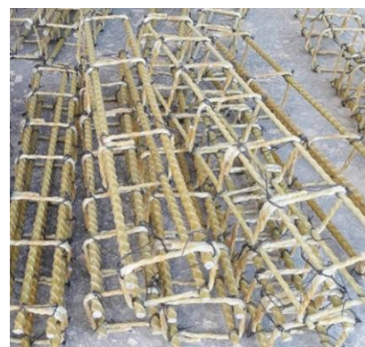
Fig. 3. Reinforcement cage for GFRP RC columns
