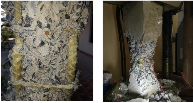
Fig. 9. Failure of the GFRP RC column specimens
