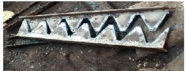
Fig. 2. Cutting of Castellated beam
