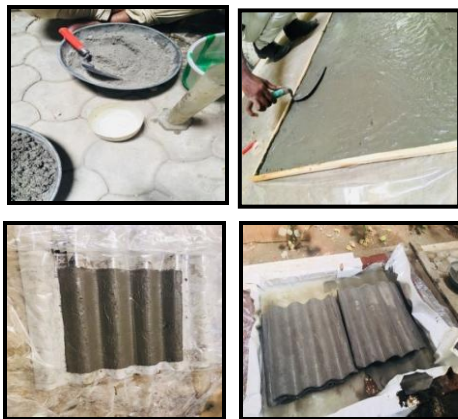
Fig1. Stages of casting corrugated sheets
