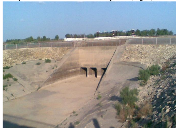
Fig. 1. The water outlet of the Mezhdurechenskoye reservoir on the downstream side
