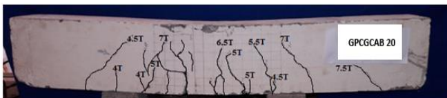
Figure XIII Crack Patterns of M 20 GPCGCA Beam
