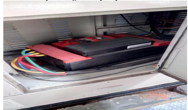
Figure 4: Cooling Tower Pump
