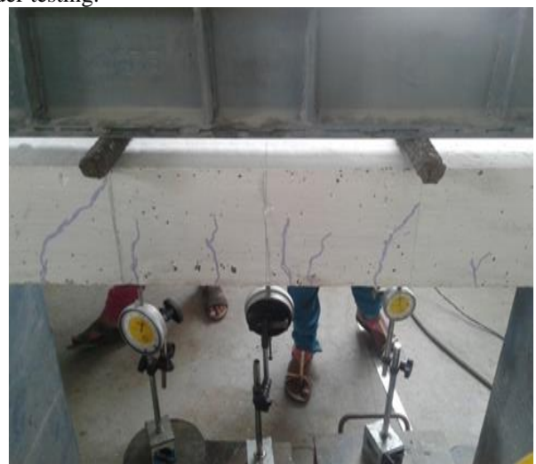
Fig 1 Crack formation in the RC Beam
