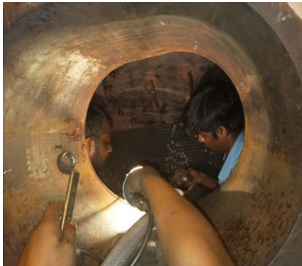
Figure – 10 Plugging of tubes
