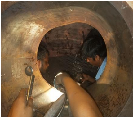
Figure – 10 Plugging of tubes
