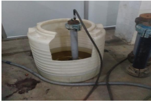
Figure 9 - Bursting Test of PVC Pipe
