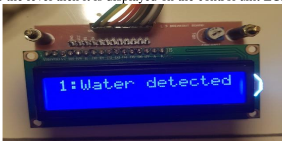
Fig.10: LCD showing water detected
