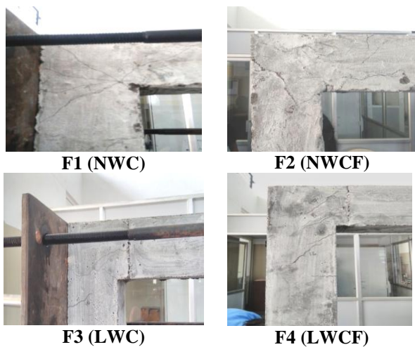
Fig. 2. Crack Patterns of Tested Specimens
