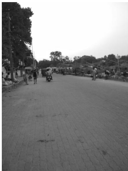
Fig. 5 Second photo showing RKM road at location A
