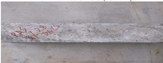
Fig (U) Failure of 3% CFRC specimen having stress of 6.55 (N/mm 2 )
