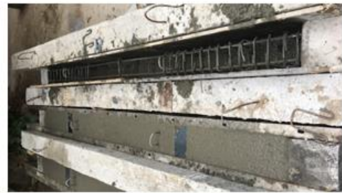
Fig. 4. Pouring the concrete layer by layer in the beams
