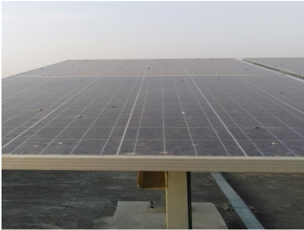
Figure 6 Shading due to Bird-Excrements
