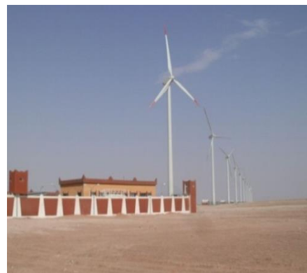
Figure 1. Wind farm G52/850, 10.2MW in Kabertene site (CDER, 2017)
