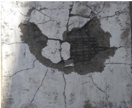
Fig 8(b): Crack pattern for GC1 slab
