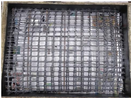
Fig 2: Arrangement of steel and geogrid
