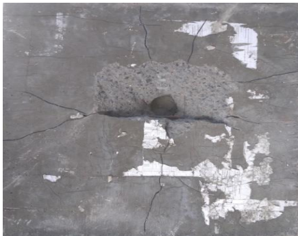
Fig 8(a): Crack pattern for RC slab
