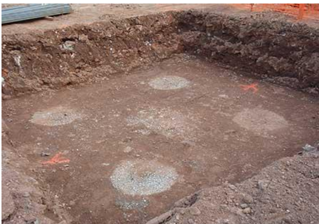
Fig. 1 Image of Stone column treated soil.
