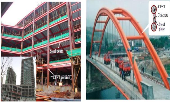
(c) Rujfeng building in Hangzhou (d) Wangcang East River Bridge
