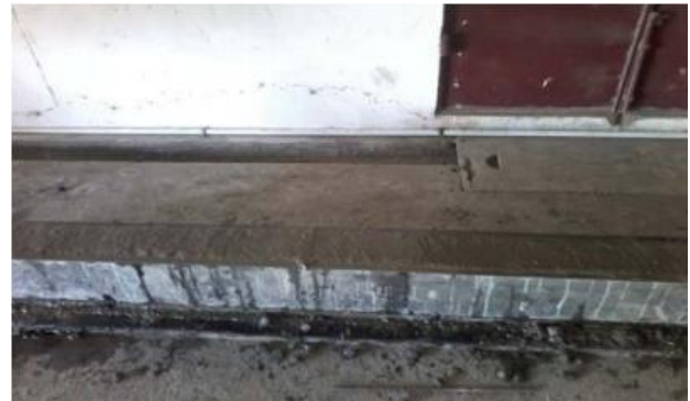
Fig 2 Casting of Beam and surface finishing
