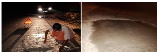
Fig. 7. Construction of WTC overlay
