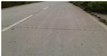
Fig. 3. Finished TWT pavement
