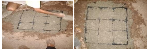
Fig. 6. Construction of CFC overlay
