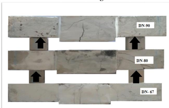
Fig. 2. Crack patterns of the retrofitted beam specimens.
