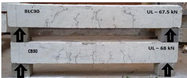
Fig 3. Crack pattern of CB30 and BLC30 beams
