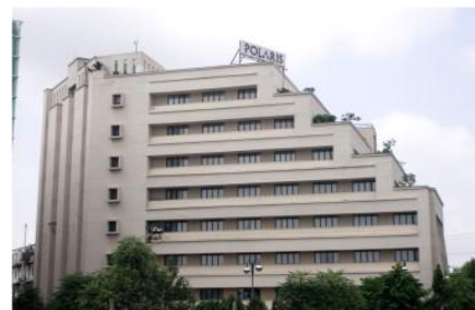
Fig. 1 Stepped building frame
