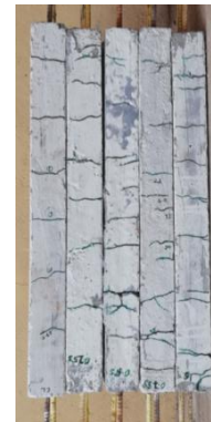
Fig 10. Crack pattern of steel fibre reinforced UHPC
