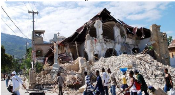
Fig.1. Failure of an URM building during 2010 Haiti earthquake [1]
