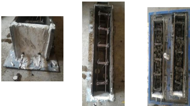
Fig 2 Preparation of moulds and pouring of concrete
