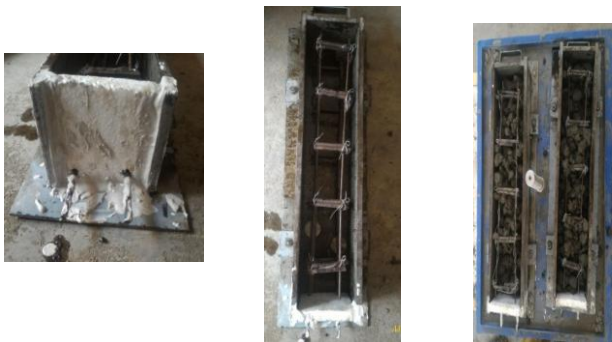
Fig 2 Preparation of moulds and pouring of concrete
