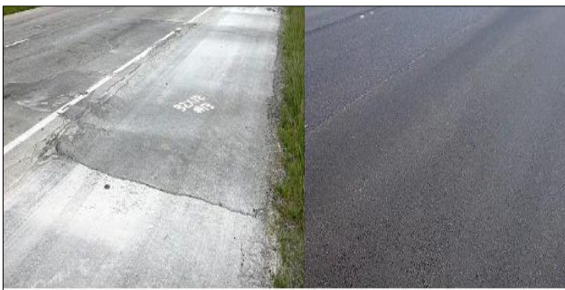
Figure 8: Road Surface Before (Left) and After (Right) Resurfacing. Amos (2006)
