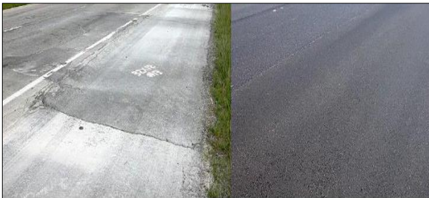
Figure 8: Road Surface Before (Left) and After (Right) Resurfacing. Amos (2006)
