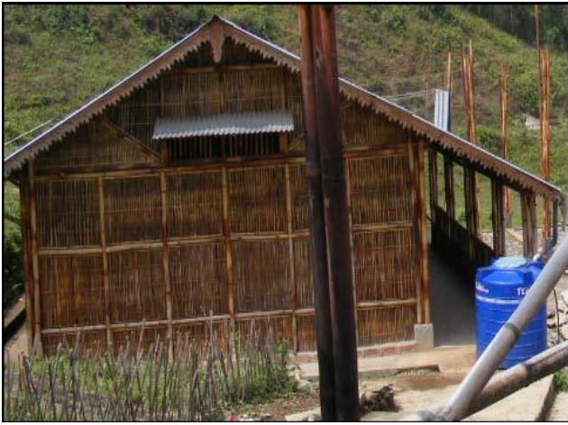
(b) a school in Darjeeling using grouted bar column base foundation
