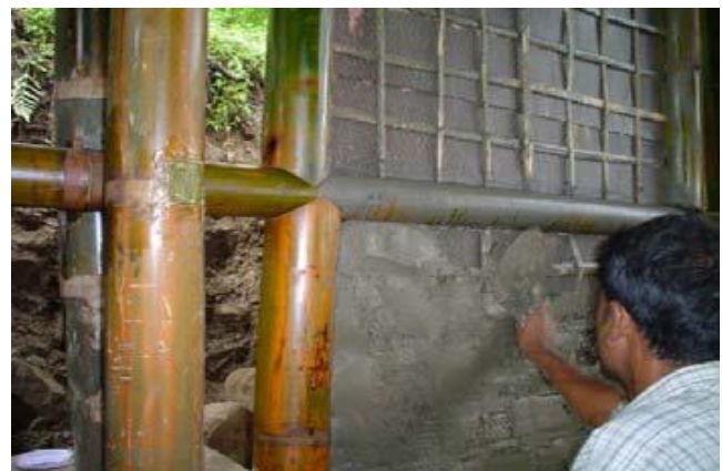
(a) Cement plastering
