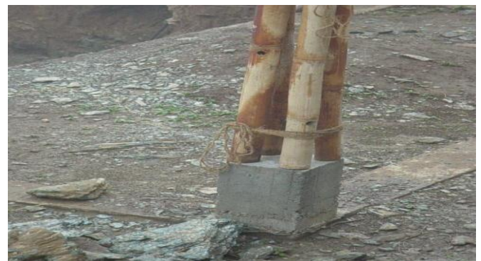
(a) grouted bar column base foundation
