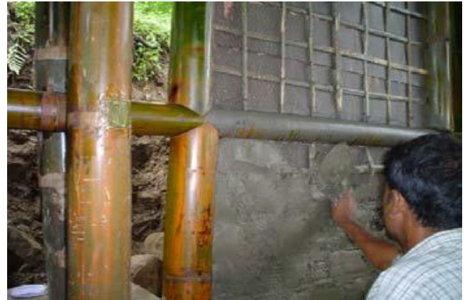
(a) Cement plastering
