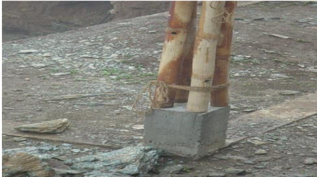
(a) grouted bar column base foundation
