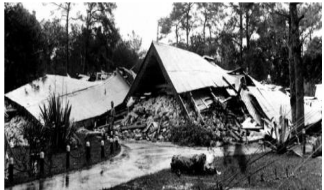
(a) The European Quarters in 1897 Shillong earthquake
