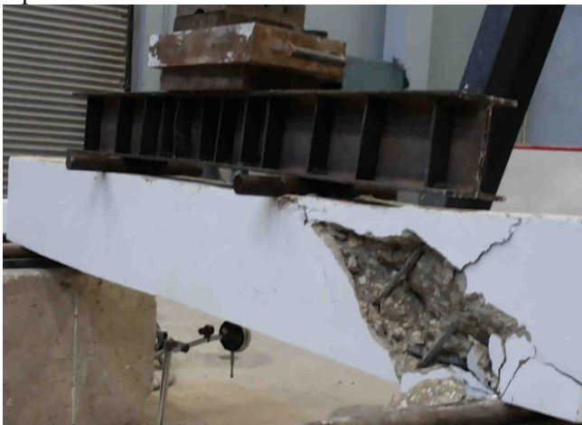
Figure 5: Typical failure mode of the beam reinforced with recycled spliced swimmer bars.
