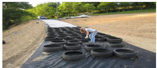
Fig 1: Laying of tire
