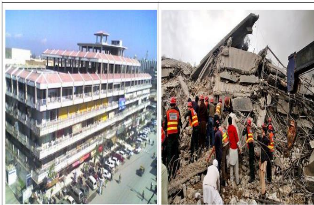
Figure15: Ghakar Plaza before and after fire incident
