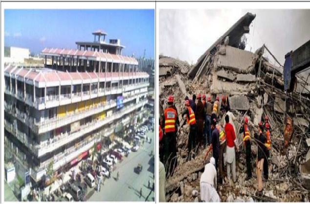
Figure15: Ghakar Plaza before and after fire incident
