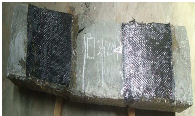
Fig. 4.5 Failure of beam H-SB1
