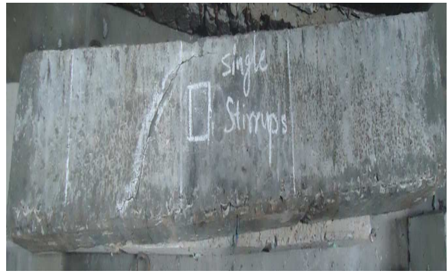
Fig. 4.3 Failure of Beam H-CB1
