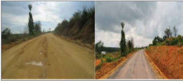
Figure 9: Before soil stabilization Figure 10: After soil stabilization (9 months after construction)
