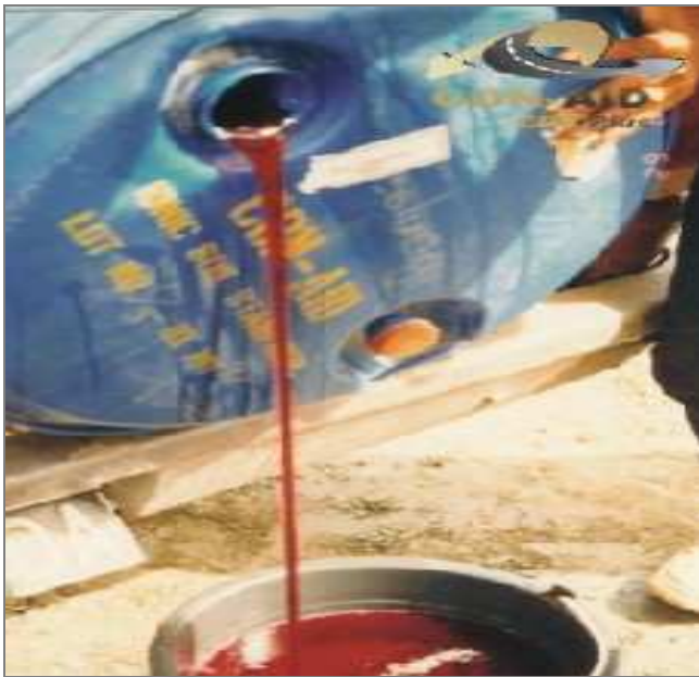
Figure 14: Con-Aid soil stabilization
