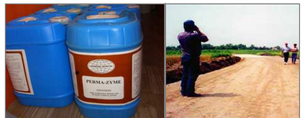
Figure 11: Perma-Zyme Soil Stabilizer and soil road using Perma-Zyme
