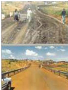
Figure 12: Phases of strength soil Figure 13: Before and after soil build-up in Con-Aid treated layers stabilization
