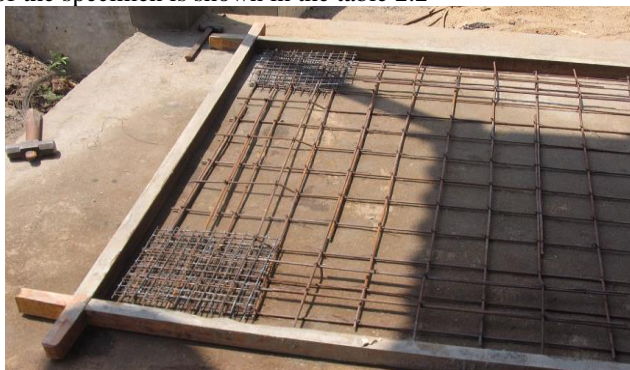
FIG.2.2. REINFORCEMENT DETAILS
