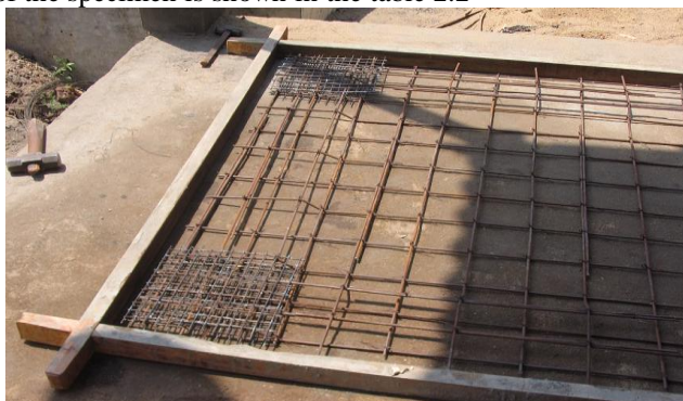
FIG.2.2. REINFORCEMENT DETAILS
