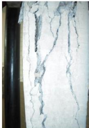
Fig. 3: Failure Pattern of Column Element CA
